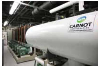
Fig. 2 Photos of the transcritical CO<sub>2</sub> system at Sobeys designed by Carnot Refrigeration.
